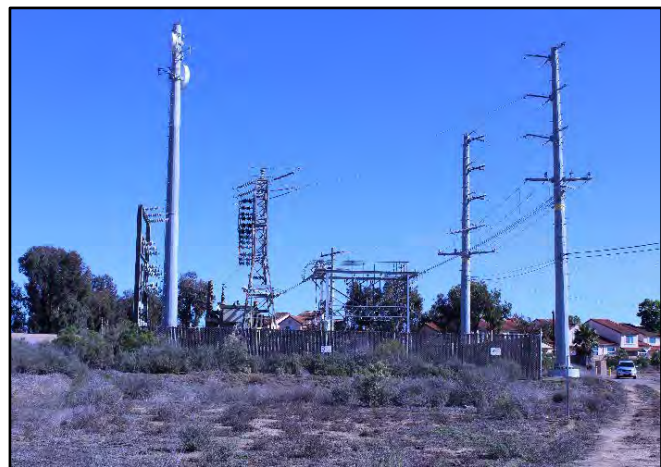
Photo 2: Stuart Mesa Substation Expansion Area (looking west)
