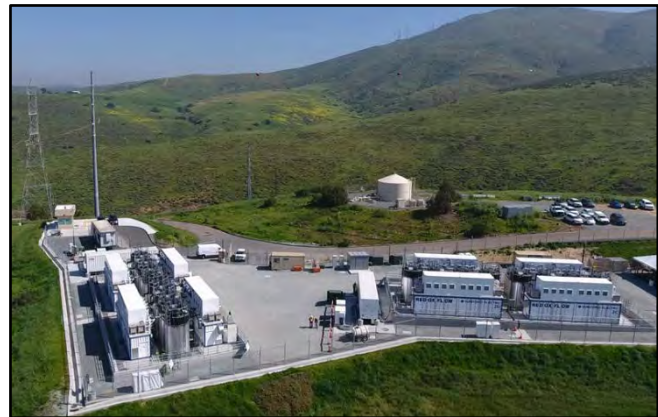
Photo 1: SDG&E Battery Energy Storage System Pilot Project (SDG&E 2019)
